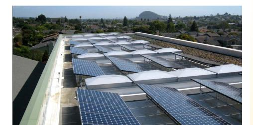
Windrush School is the first LEED Platinum school building in California. The roof of the Library/Middle School Building features both a solar array and a living roof which provides for increased insulation, decreased energy demands for cooling and heating and support for bird and insect life.
