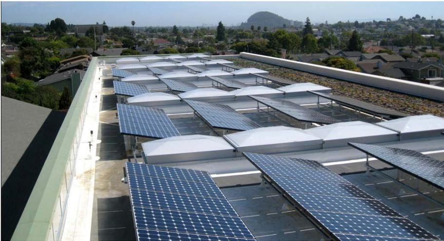
**Windrush School is the first LEED Platinum school building in California.** The roof of the Library/Middle School Building features both a solar array and a living roof which provides for increased insulation, decreased energy demands for cooling and heating and support for bird and insect life.
